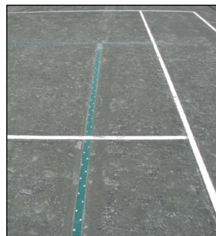
Full-size (78') Clay Court with Permanent Nail Down Shared Lines: Charlottesville, Virginia
